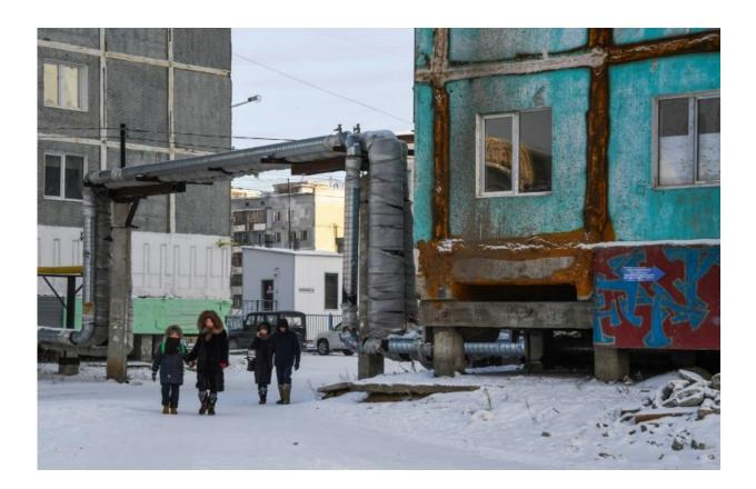
Many houses in Yakutsk are made up of concrete panels and stand on stilts which ensure ventilation of the building's underbelly and prevent it from heating the permafrost, the layer of mineral cemented together with water which is stable as long as it stays frozen. But warmer temperatures are threatening that
