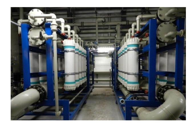
An ultrafiltration system consists of extremely fine membrane sections, in which antibiotics-resistant bacteria are removed from the sewage. Credit: HyReKA
