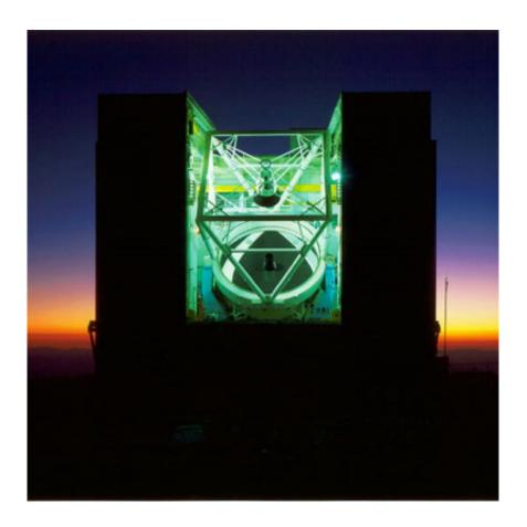
The MMT Telescope is located on Mount Hopkins, 47 miles south of Tucson. When the telescope was completed in 1979, it was called the Multiple-Mirror Telescope, as it was comprised of six smaller mirrors. The smaller mirrors were replaced by a single 6.5-meter mirror in 2000, but the name MMT was retained. Credit: Courtesy of the MMT Observatory
