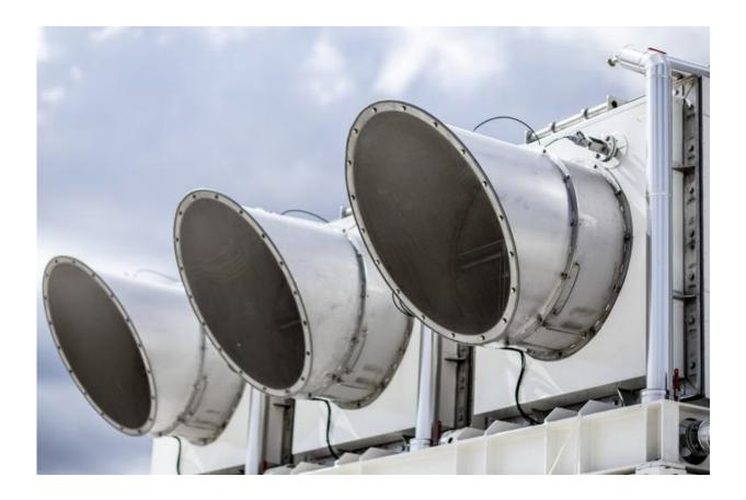
A handful of commercial companies are testing direct air capture technology,, which takes carbon dioxide out of the air. This project in Italy will use the CO2 to ultimately produce natural gas to power vehicles. Credit: <u>Climeworks</u>
