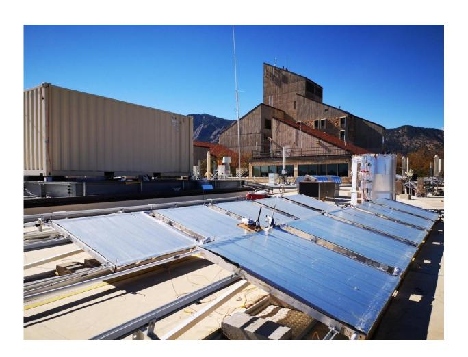
An array of RadiCold cooling modules on the roof of a building on the University of Colorado Boulder campus. Credit: Yang Lab / University of Colorado Boulder
