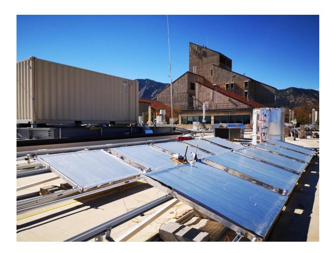
An array of RadiCold cooling modules on the roof of a building on the University of Colorado Boulder campus. Credit: Yang Lab / University of Colorado Boulder
