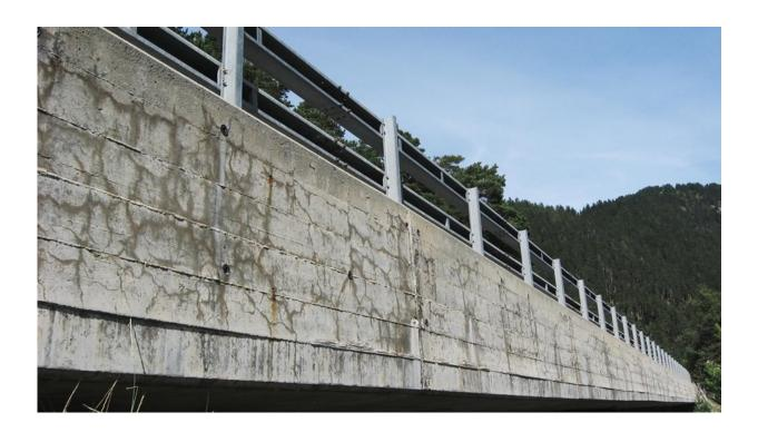
Concrete structures that have been damaged by AAR (alkali-aggregate reaction) exhibit these typical cracks. The dark color around the edges of the cracks is caused by leaking AAR products. Credit: Swiss Federal Laboratories for Materials Science and Technology
