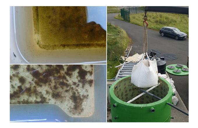
Water-flea-based filters (left) could be combined with earthworm-based systems (right) to treat wastewater. Credit: INNOQUA
