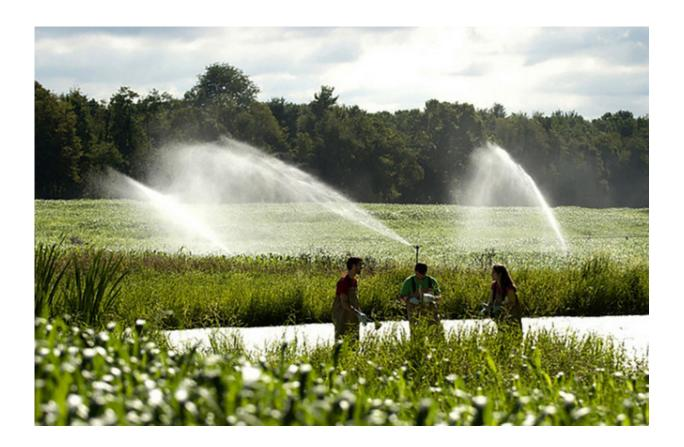
Penn State's Living Filter is a 50-year-old wastewater reuse system that sprayirrigates treated effluent from the University Park campus's sewage treatment plant on 600 acres of farm and forest. Unique in the eastern United States, the facility provides opportunities for researchers to conduct a wide range of water-quality experiments. Credit: Penn State
