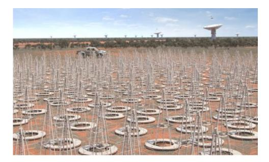
The SKA will have over 2000 radio dishes and 2 million low-frequency antennas once finished. Credit: The Square Kilometre Array
