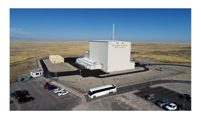
INL's Transient Reactor Test Facility (TREAT) exposes nuclear fuel to extreme, accident-like conditions to provide valuable data that researchers and industry use to develop more robust fuels. Credit: Idaho National Laboratory
