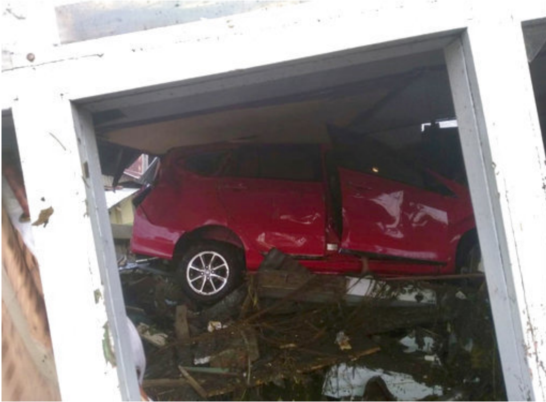
A car swept away by tsunami is seen stuck under a damaged building in Palu, Central Sulawesi, Indonesia, Saturday, Sept. 29, 2018. A powerful earthquake rocked the Indonesian island of Sulawesi on Friday, triggering a 3-meter-tall (10-foot-tall) tsunami that an official said swept away houses in at least two cities. (Dede Budiarto via AP)
