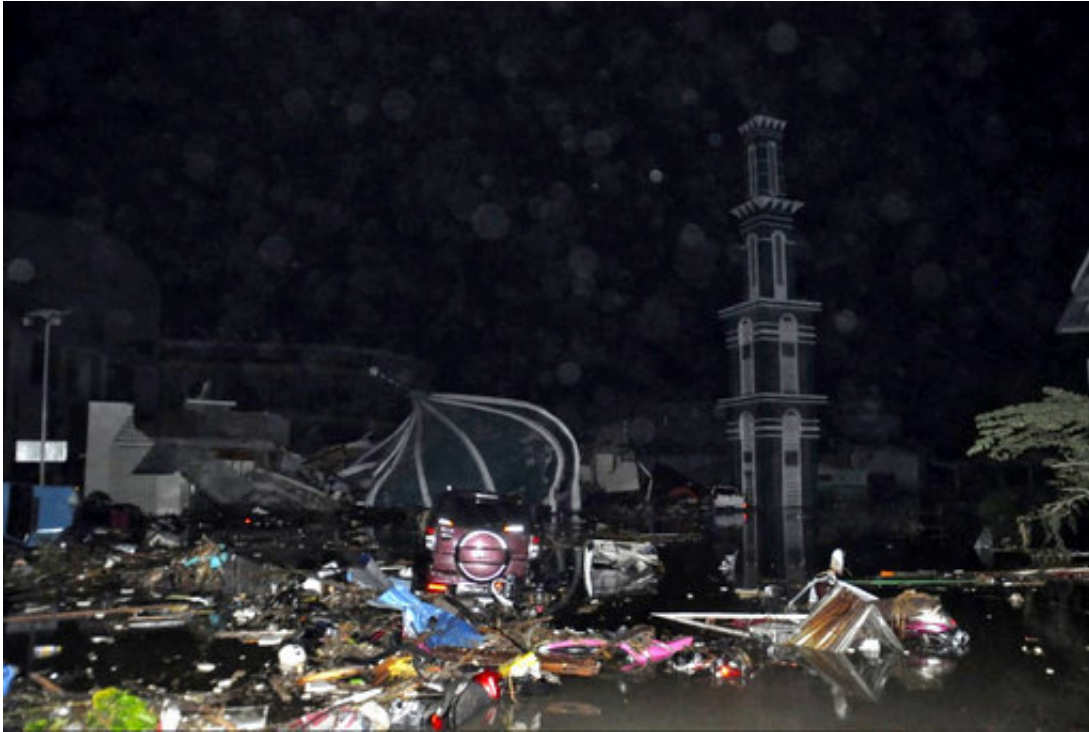
A mosque is seen heavily damaged by earthquake and tsunami in Palu, Central Sulawesi, Indonesia, Saturday, Sept. 29, 2018. The powerful earthquake rocked the Indonesian island of Sulawesi on Friday, triggering a 3-meter-tall (10-foot-tall) tsunami that an official said swept away houses in at least two cities. (AP Photo/Rifki)
