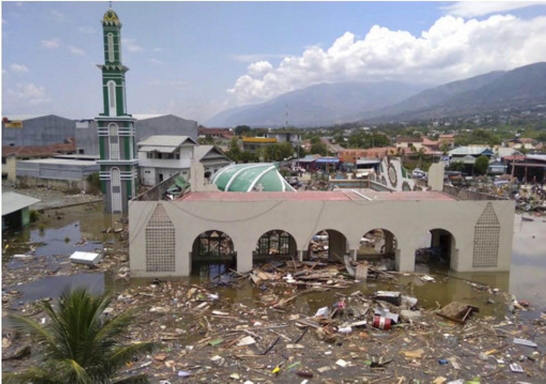
The ruin of a mosque badly damaged by earthquake and tsunami is seen in Palu, Central Sulawesi, Indonesia, Saturday, Sept. 29, 2018. The powerful earthquake rocked the Indonesian island of Sulawesi on Friday, triggering a 3-meter-tall (10-foot-tall) tsunami that an official said swept away houses in at least two cities. (AP Photo/Rifki)
