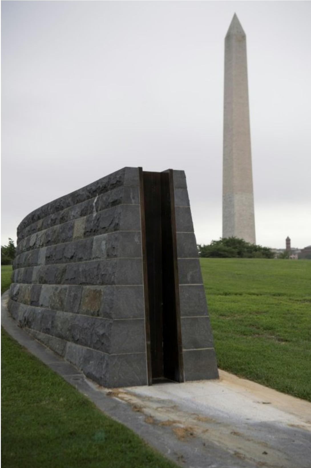
The Potomac Park Flood Levee sits a stone's throw from the White House and
