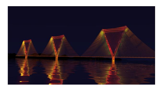
Split-pylon concept bridge to cross Strait of Gibraltar, with two 5km main spans. Credit: Helen Fairclough
