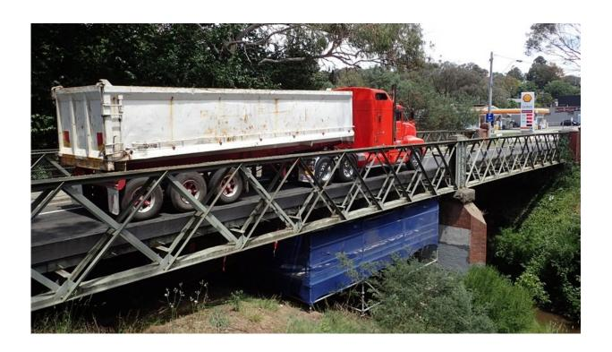
The Diamond Creek Bridge near Melboune was reinforced with CFRP strips in 2018 and tested for durability with a 42-ton truck after work. Credit: Swiss Federal Laboratories for Materials Science and Technology
