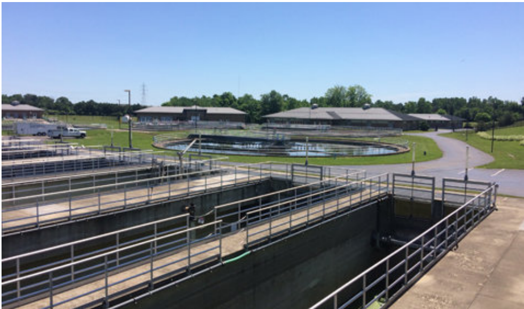
Alum Creek Waste Water Reclamation Facility. Credit: Ohio University
