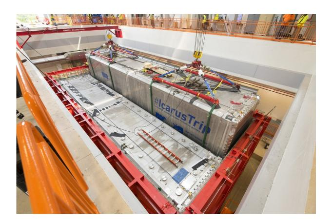
The second of two ICARUS detector modules is lowered into its place in the detector hall. Credit: Reidar Hahn
