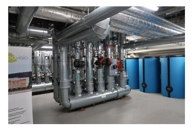
The aquifer storage system in Bonn supplies up to 80% of the heat and cold in three buildings covering a total area of 60,000 m<sup>2</sup>. Credit: Paul Fleuchaus, KIT
