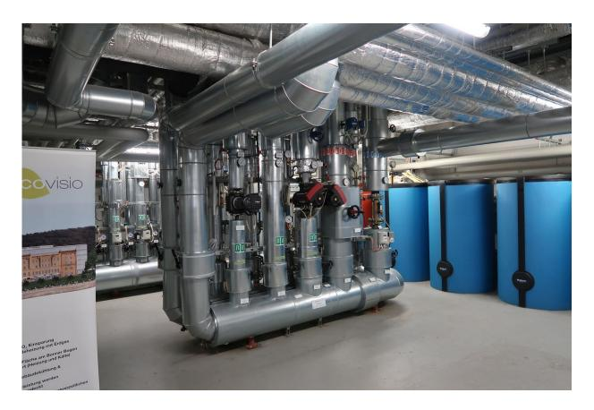
The aquifer storage system in Bonn supplies up to 80% of the heat and cold in three buildings covering a total area of 60,000 m<sup>2</sup>. Credit: Paul Fleuchaus, KIT
