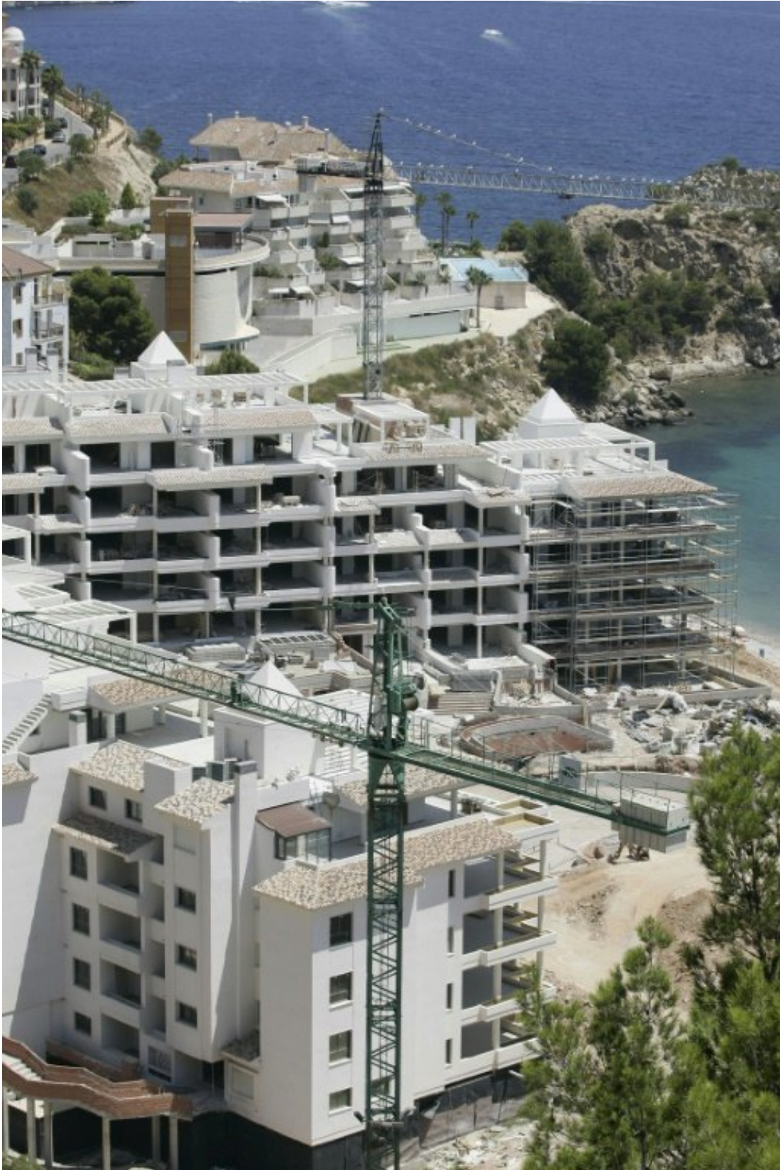
Construction work in Altea on Spain's Costa del Sol, pictured July 29, 2007
