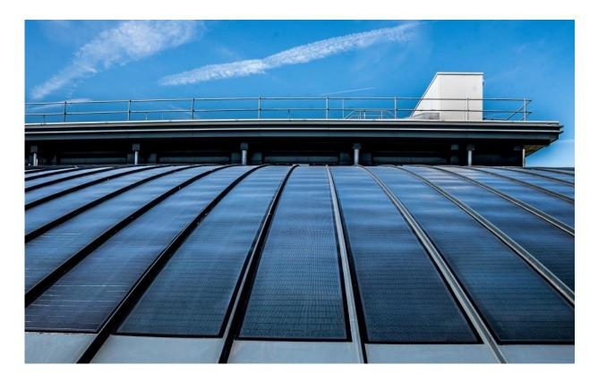
This is on the Active Office, one of two energy-positive buildings designed by a Swansea University-led research team. The photovoltaic cells are integrated into the roof. And the panels are flexible, which extends their uses. Credit: SPECIFIC/Swansea University
