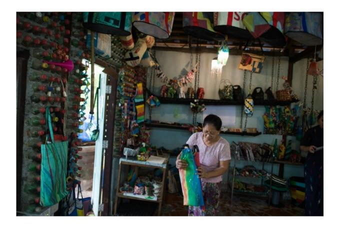
Even the shop is made from reused waste, with walls formed by cemented plastic bottles and a roof made from old tyres
