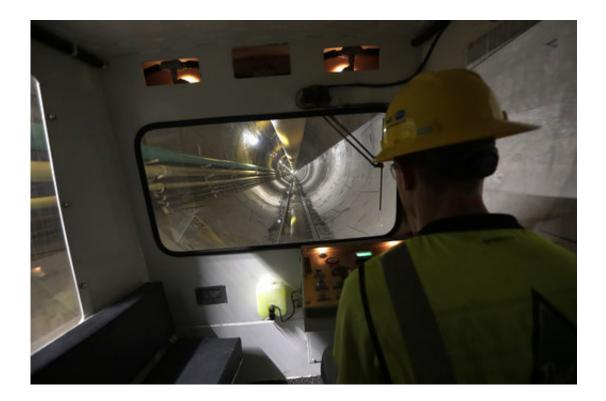
In this Wednesday, May 16, 2018 photo, operator Andrew Reisinger drives a personnel shuttle along a small gauge rail line inside a 2.5-mile bypass tunnel being dug for the Delaware Aqueduct, in Marlboro, N.Y. Hard-hat workers are toiling deep underground, 55 stories beneath the Hudson River, to eliminate gushing leaks in an aging tunnel that carries half the city's water supply over 85 miles from Catskill Mountain reservoirs. (AP Photo/Julie Jacobson)
