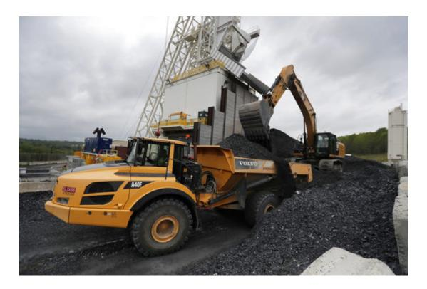
In this Wednesday, May 16, 2018 photo, an excavator loads a dump truck with shale from a 2.5-mile bypass tunnel being dug for the Delaware Aqueduct, in Marlboro, N.Y. Hard-hat workers are toiling deep underground, 55 stories beneath the Hudson River, to eliminate gushing leaks in an aging tunnel that carries half the city's water supply over 85 miles from Catskill Mountain reservoirs. (AP Photo/Julie Jacobson)
