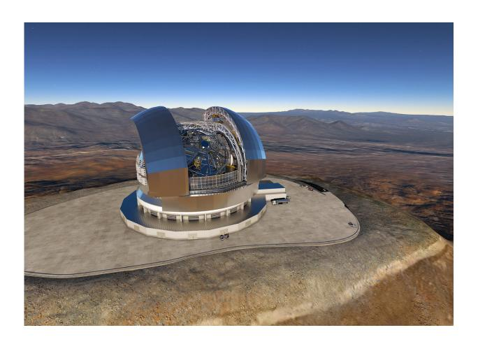
In Chile, the European Southern Observatory ESO is building the Extremely Large Telescope (ELT) with a mirror diameter of 39 meters. Credit: ESO/L. Calçada/Ace Consortium
