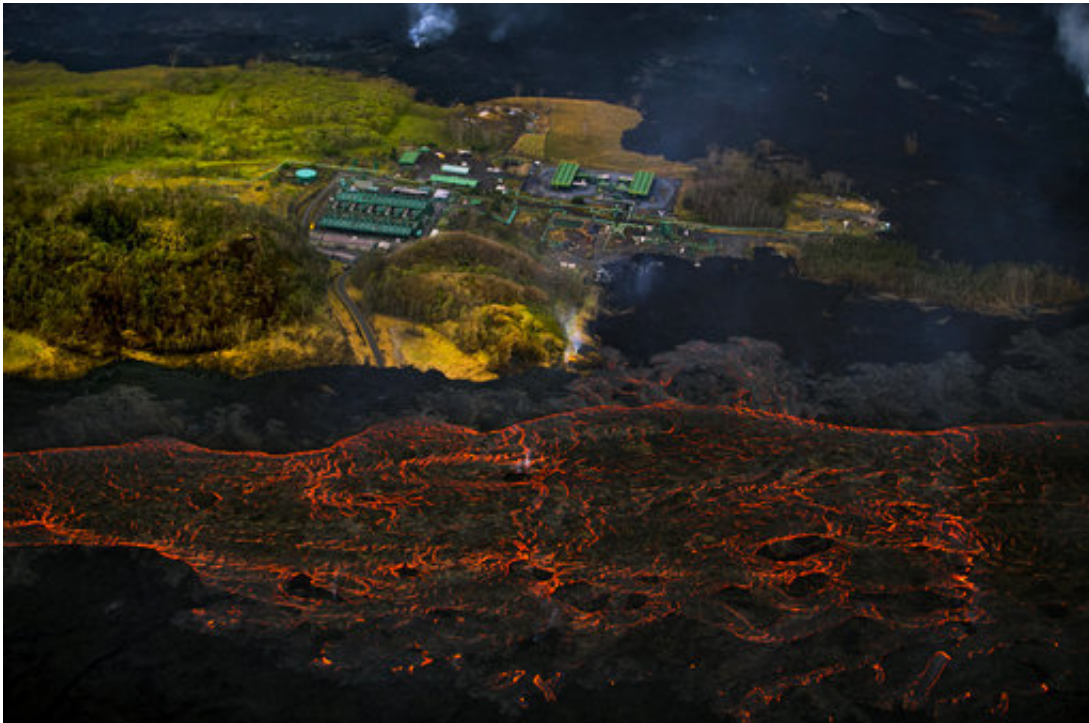
Lava from the Kilauea volcano flows near the Puna Geothermal Venture power plant on Sunday, June 10, 2018, in Pahoa, Hawaii. (AP Photo/L.E. Baskow)
