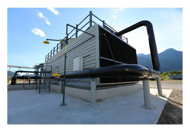
Carbon Engineering's pilot air contactor, constructed from the same set of cooling tower componentry and design philosophy that will be used at commercial scale. Credit: Carbon Engineering
