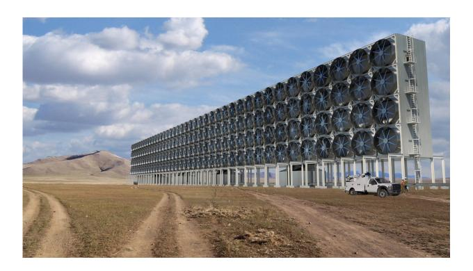
This rendering shows Carbon Engineering's proposed air contactor design. This unit would be one of several that would collectively capture 1M tons of CO2 per year. Credit: Carbon Engineering
