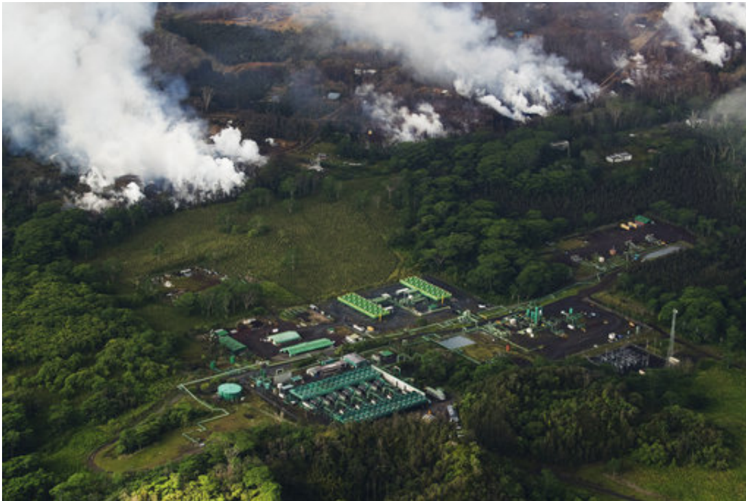
An aerial view of Hawaii's Kilauea East Rift zone and the Puna Geothermal Venture plant is seen, Wednesday, May 16, 2018. Earthquakes were damaging roads and buildings on Hawaii's Big Island on Wednesday as ash emissions streamed from Kilauea volcano. (Cindy Ellen Russell/Honolulu Star-Advertiser via AP)
