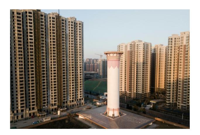
Standing between high-rises, the giant air purifier is capable of cleaning between 5 million and 18 million cubic meters of air each day, depending on the weather, season, and level of pollution, according to a report by a Chinese website
