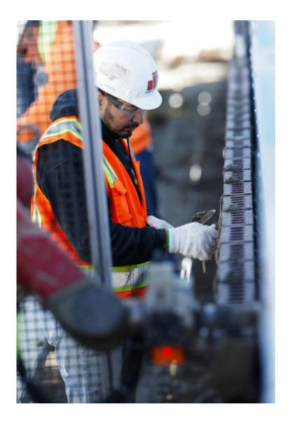
In this Tuesday, Feb. 27, 2018, photo, a mason completes finishing work as he follows Samantha, a robotic bricklayer, at work on the facade of a school in the south Denver suburb of Englewood, Colo. Faced with a shortage of skilled laborers, construction industry leaders hope that robots—and other technologies—can be used to boost productivity, workplace safety and speed in building housing and infrastructure in the decades ahead. (AP Photo/David Zalubowski)
