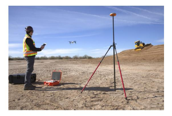
In this undated photo provided by Kespry, a Kespry drone is used to measure earthwork grading operations on a construction site. Robots are coming to a construction site near you. Tech startups are developing self-driving bulldozers, survey drones and bricklaying robots to help the construction industry boost productivity, speed and safety as it struggles to find enough skilled workers. (Adam Crowley/Kespry via AP)
