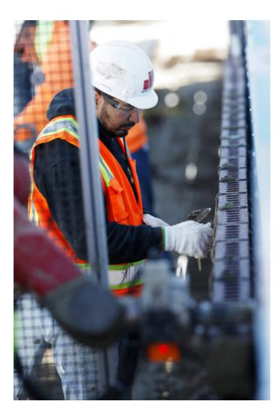
In this Tuesday, Feb. 27, 2018, photo, a mason completes finishing work as he follows Samantha, a robotic bricklayer, at work on the facade of a school in the south Denver suburb of Englewood, Colo. Faced with a shortage of skilled laborers, construction industry leaders hope that robots—and other technologies—can be used to boost productivity, workplace safety and speed in building housing and infrastructure in the decades ahead. (AP Photo/David Zalubowski)
