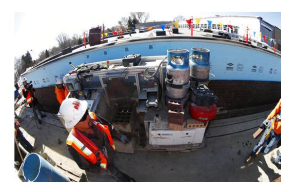
In this Tuesday, Feb. 27, 2018, photo taken with a fisheye lens, Samantha, a robotic bricklayer, is shown at work on the facade of a school in the south Denver suburb of Englewood, Colo. Faced with a shortage of skilled labor, the construction industry hopes that robots and other technologies will help boost productivity, safety and speed to build more housing and deal with infrastructure needs in the decades ahead. (AP Photo/David Zalubowski)
