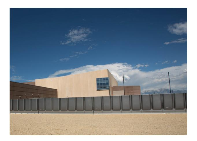
A row of fuel cells (in the foreground) power an eBay data center near Salt Lake City. Similar fuel cells could be more efficient -- and commonplace -incorporating new materials in development by UW-Madison engineers. Credit: Bloom Energy
