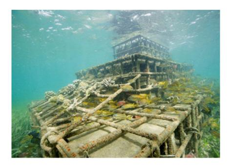
Pilot structures installed in Grenville Bay, Granada, can provide protection from coastal erosion and help to restore degraded coral reefs. Credit: Tim Calver
