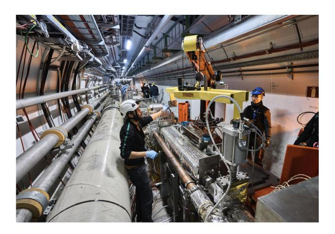
Installation of a collimator in the LHC. Collimators protect the sensitive equipment from escaping particles. Credit: Maximilien Brice, Julien Ordan/CERN
