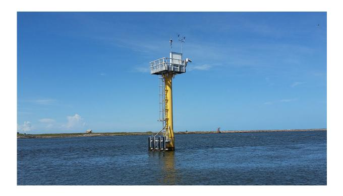
A tide level gauge that has been bolstered to withstand hurricanes. Researchers have shown that sea-level rise is changing patterns of the tides in the Delaware and Chesapeake bays. Credit: NOAA
