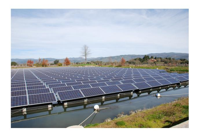
A floatovoltaic installation at Far Niente Winery in Oakville, Calif., comprises nearly 1,000 solar panels floating on pontoons on the vineyard irrigation pond. Credit: Far Niente Winery
