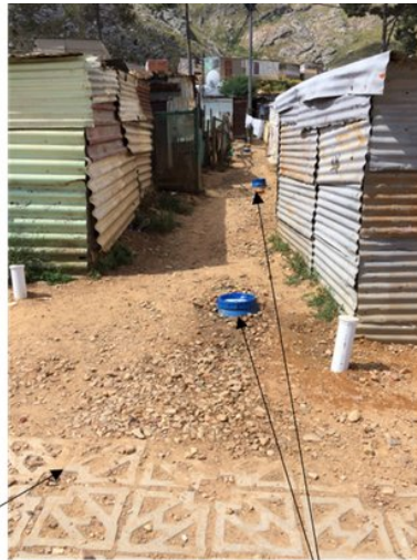
Greywater disposal points
