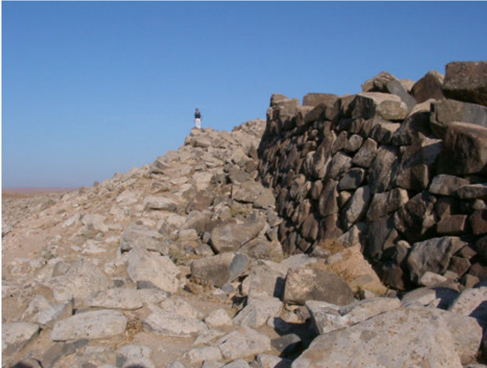
Access ramp at Qal'at al-Rahiyya, view toward the northwest. Credit: M.-O. Rousset mission Marges arides
