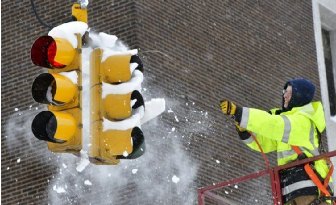
City of Erie traffic engineering employee Chuck Carnes Jr. uses compressed air to clear snow from a traffic signal in Erie, Pa., Wednesday, Dec. 27, 2017. Carnes was part of a two-man crew clearing signals after a record-setting snowfall. (Greg Wohlford/Erie Times-News via AP)
