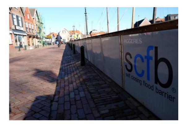
In this Nov. 6, 2017, photo, a man rides a bicycle next to self-raising dike n in the Dutch fishing village of Spakenburg, Netherlands. The 300-meter long dike that is raised by the very flood waters it is designed to hold back is an example of Dutch ingenuity in flood prevention that is becoming a major export earner for this low-lying nation. (AP Photo/Mike Corder)
