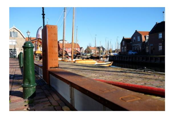
In this Nov. 6, 2017, photo, a self-raising dike is seen in the Dutch fishing village of Spakenburg. The 300-meter long dike that is raised by the very flood waters it is designed to hold back is an example of Dutch ingenuity in flood prevention that is becoming a major export earner for this low-lying nation. (AP Photo/Mike Corder)
