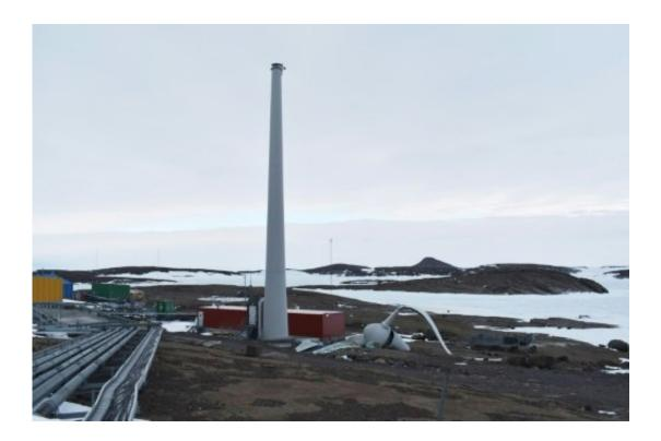
The head of a wind turbine lies on the ground at Australia's Antarctic Division's Mawson station after it broke off narrowly missing a storage building
