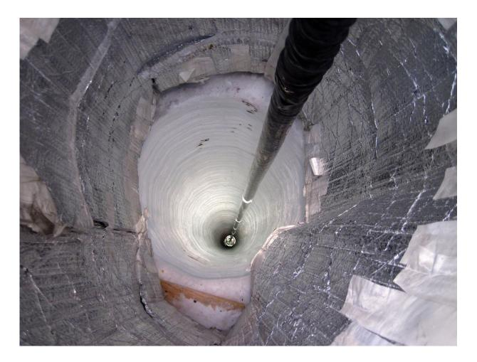
A cable with a string of neutrino decectors being lowered down into one of the deep holes in the ice near the South Pole during the installation of the IceCube telescope. Credit: NSF/B.Gudbjartsson
