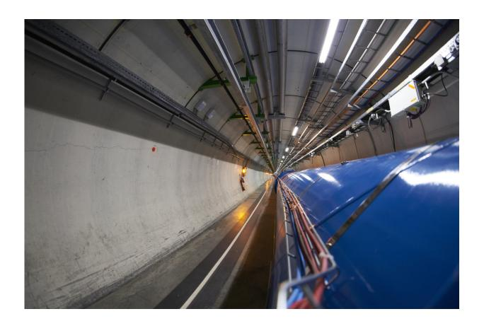
Trillions of protons race around the LHC's 27km ring in opposite directions more than 11,000 times a second, travelling at 99.999991 per cent the speed of light. Credit: Max Brice and Julien Ordan/CERN
