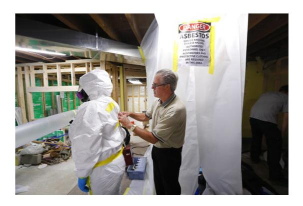
In this Oct. 18, 2017, photo, George Riegel, Jr., M.D., right, owner of Asbestos Removal Technologies Inc., helps prepare a personal air monitor on job forman Megan Eberhart before asbestos abatement in Howell, Mich. Congress ordered the EPA review last year to gauge risks of asbestos and nine other highly toxic substances and find better ways to manage them for public safety. (AP Photo/Paul Sancya)
