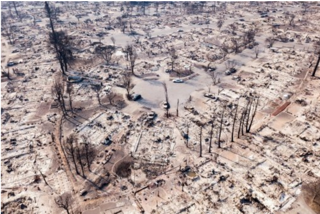
Fire damage in the Coffey Park neighborhood of Santa Rosa, California
