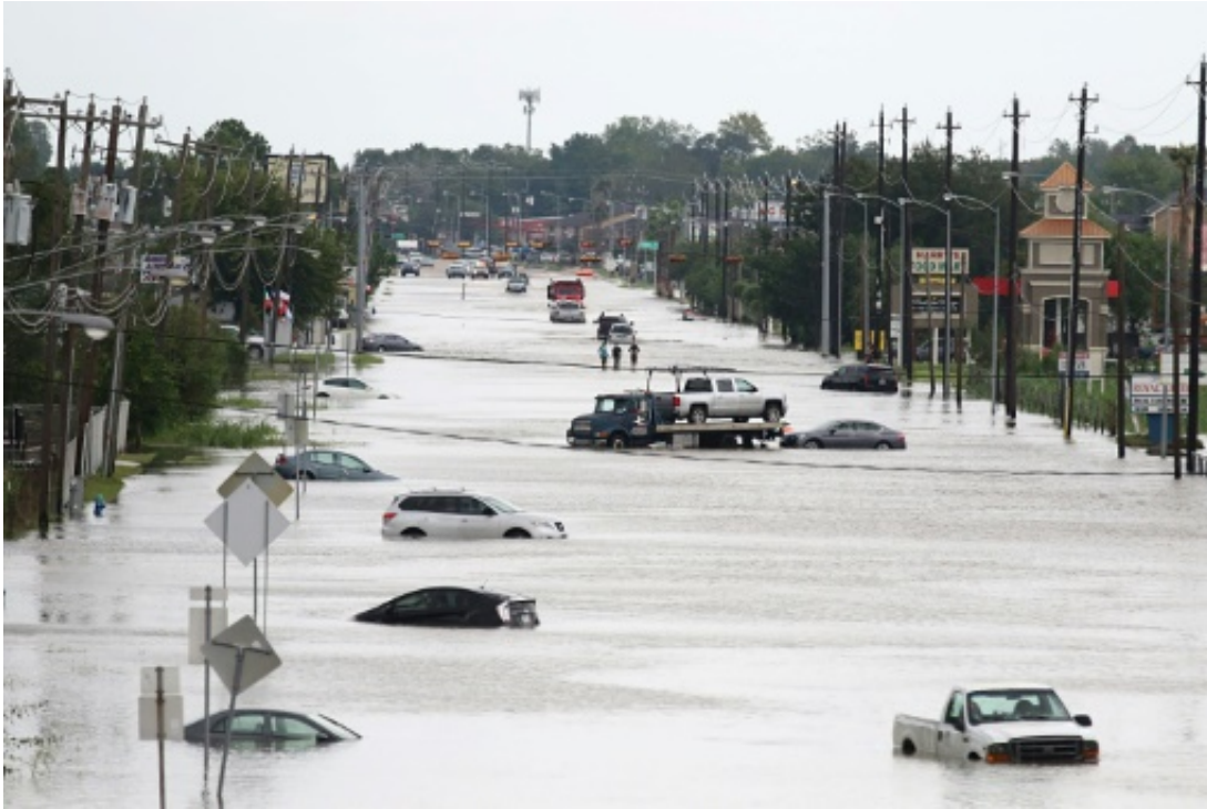
Floodwaters on Telephone Road in Houston on August 30
