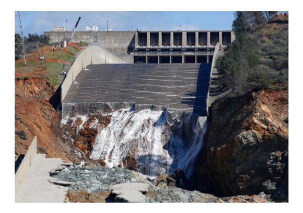
In this Feb. 28, 2017, file photo, water flows down the Oroville Dam's crippled spillway in Oroville, Calif. An independent team of dam experts says bad design and construction a half-century ago contributed to a disastrous spillway collapse at the nation's tallest dam. Dam-safety experts investigating February's spillway failures at the Oroville Dam say California should have assessed the original flaws. (AP Photo/Rich Pedroncelli, File)
