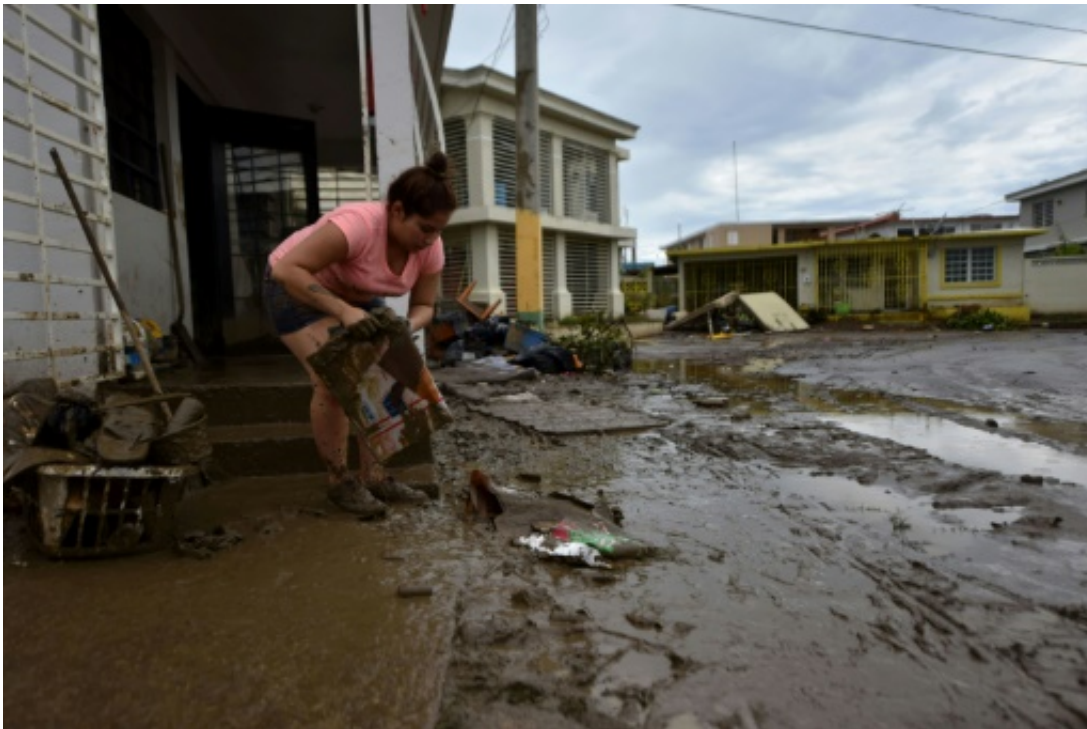
A woman removes mud from her damaged house in Toa Baja, near San Juan, Puerto Rico
