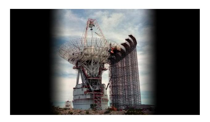
In order to "talk" with the distant Voyager spacecraft, NASA had to leap forward in space communication technology. In the image above, a 64-meter-wide antenna dish in Goldstone, Calif. is expanded to 70 meters. Credit: NASA/JPL-Caltech
