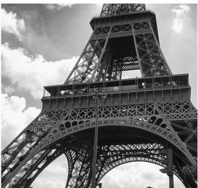
The intricate skeleton of Euplectella aspergillum (left), and the Eiffel Tower (right). Both structures are composed of an assembly of beam-like elements. Credit: Michael A. Monn, CC BY-ND
