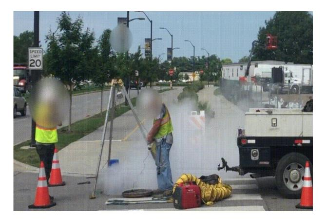
Workers repair a damaged pipe using the CIPP process, which emits a white plume containing a complex mixture vapors and chemical droplets. The workers wore no respiratory protection. Credit: Purdue University
