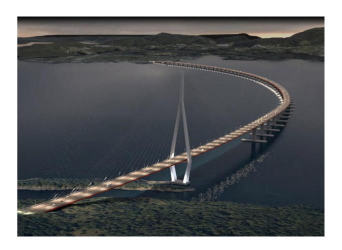
Illustration of the floating bridge across the Bjørnafjord. The distance to the first pontoon is more than 400 metres, which is more or less the same length as the main span of the Lysefjord bridge. Credit: SVV / Vianova / Baezeni
