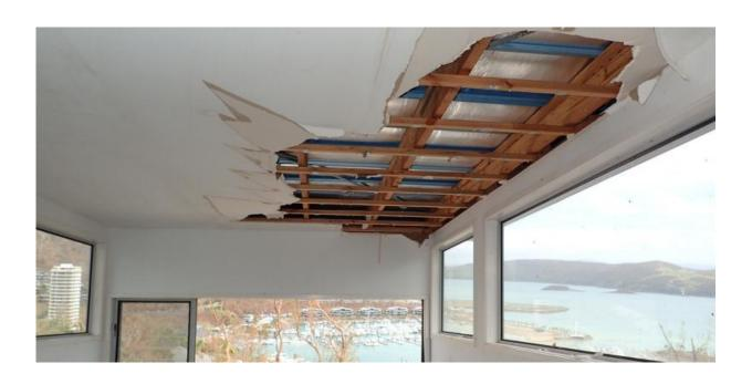
The none-structural storm damage: ceiling failure due to water ingress into roof cavity. Author provided
