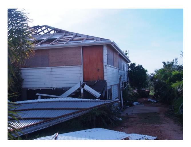
Loss of roofing due to a batten to rafter failure in a pre 1980s home where wind speeds were less than 80% of design.
